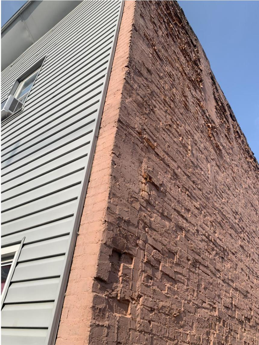
**1:** Wall is considered plumb with severe brick erosion present
