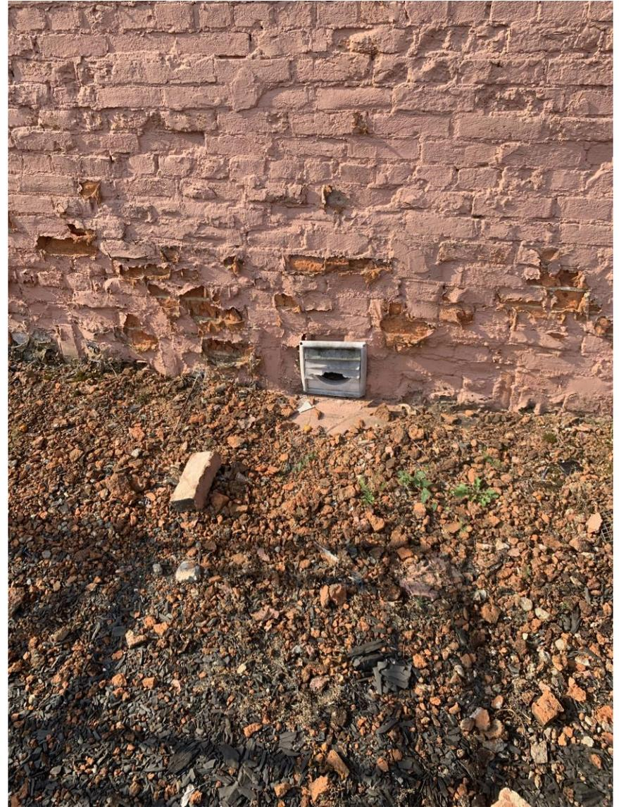
**8:** Vent extends through wall; Wall construction consists of header & stretcher coursing indicating that this is a bearing wall
