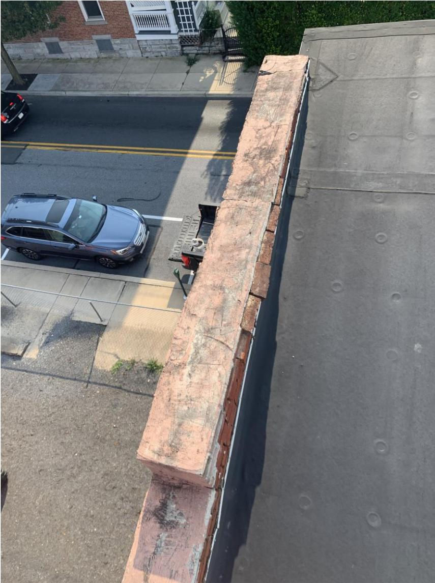
**13:** Exposed brick face has dislodged brick about to fall on adjacent roof
