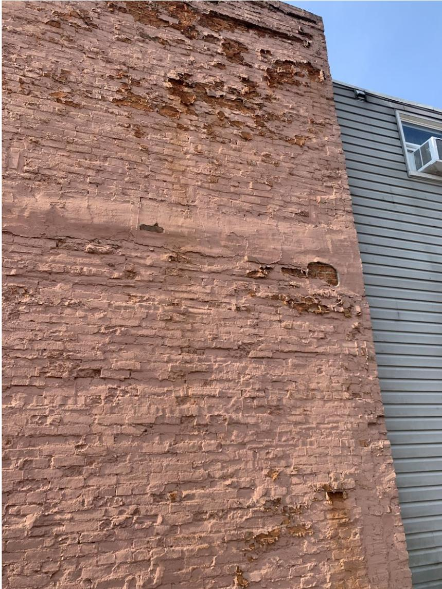
**21:** Wall has apparent filled in joist pockets from building that was removed
