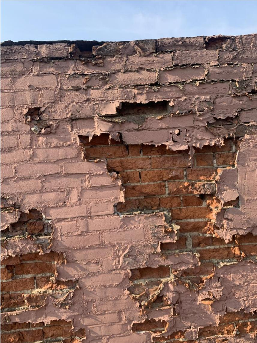
**11:** Painted surface has deteriorated and allowed moisture & erosion damage to occur
