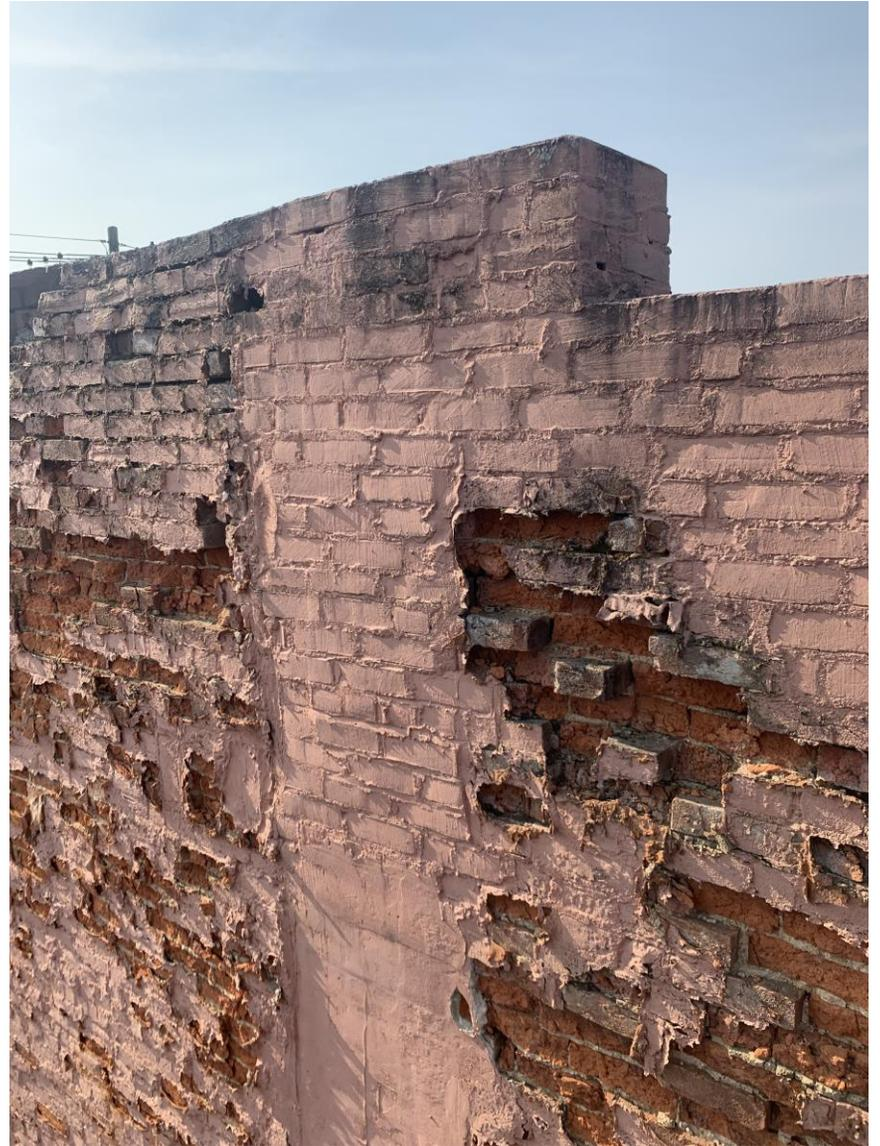
**12:** Painted surface has deteriorated and allowed moisture & erosion damage to occur
