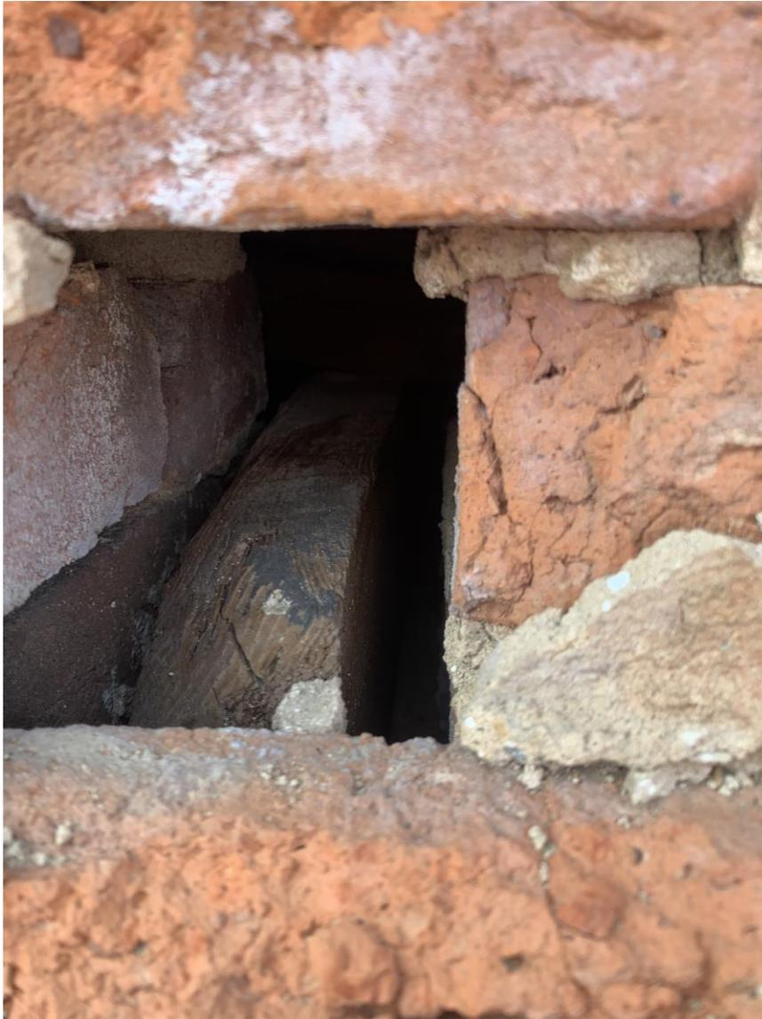
**17:** Close-up of joist support of adjacent building's roof
