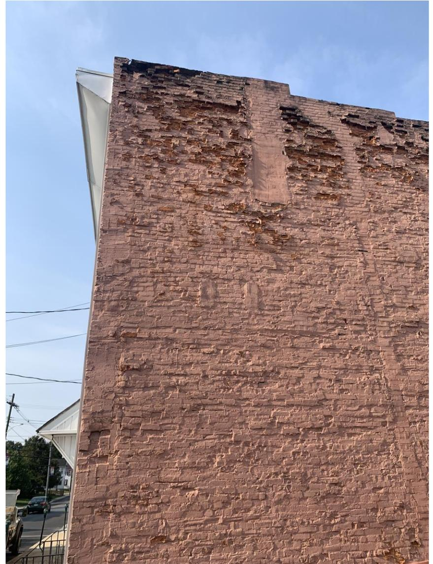
**2:** Wall has evidence of previous repairs at a chimney, intersecting wall, and joist support pockets
