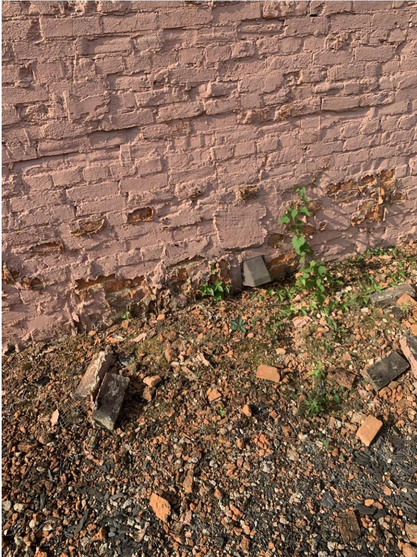
**7:** Vent extends through wall; Wall construction consists of header & stretcher coursing indicating that this is a bearing wall
