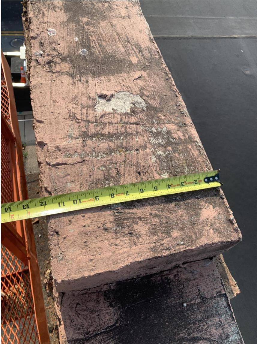
**19:** Wall thickness is 12” and consists of (3) wythes of brick
