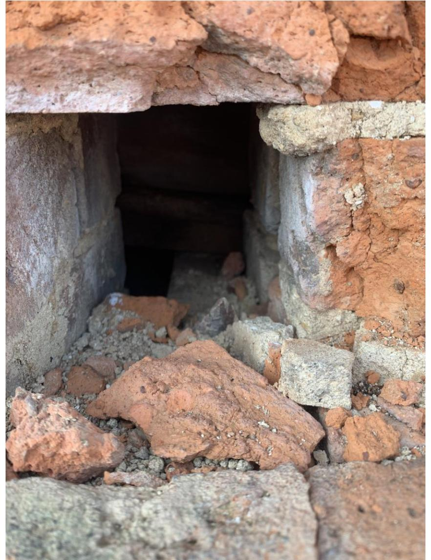
**18:** Close-up of joist support of adjacent building's roof
